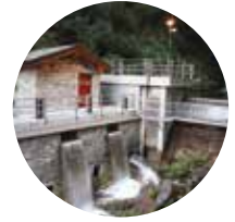
HYDRO POWER PLANTS
